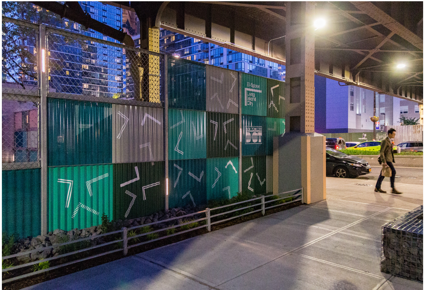
EI-Fence with integrated lighting at Dutch Kills Street and Jackson Avenue in Long Island City, Queens (NYC Department of Transportation)
