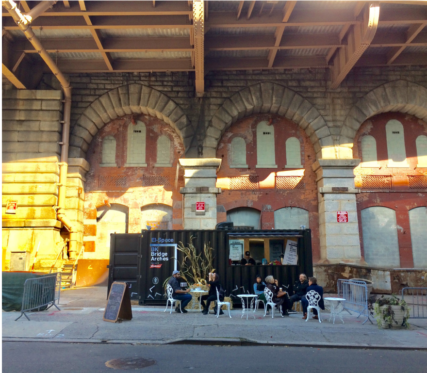
El-Box located under the south side of the Brooklyn Bridge in Lower Manhattan (NYC Department of Transportation)
