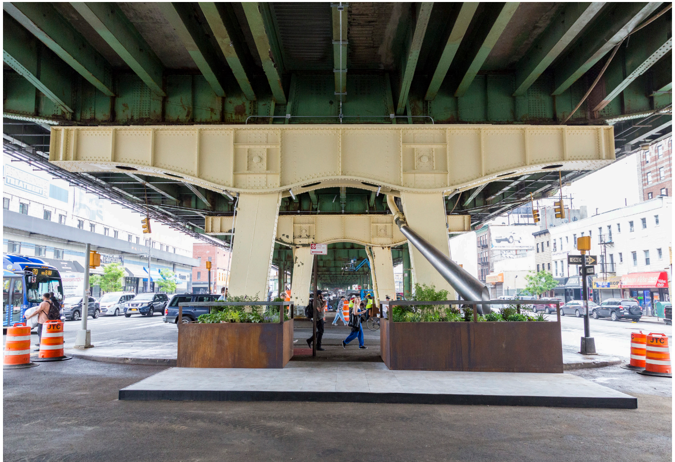
Above grade planters capturing stormwater through a cone downspout in Sunset Park, Brooklyn (NYC Department of Transportation)
