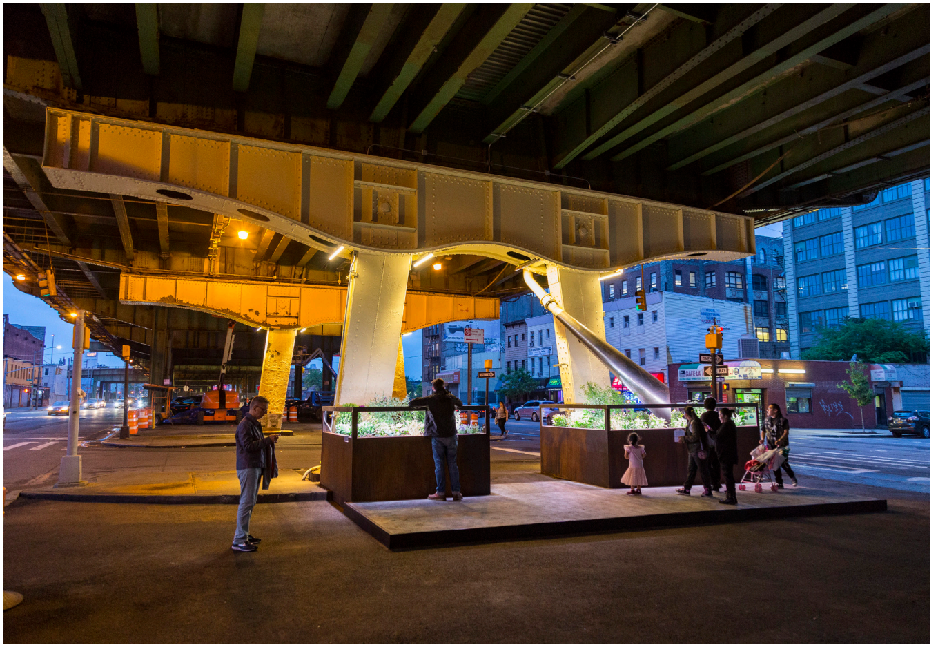
Lighting improvements at the intersection of 36th Street and 3rd Avenue in Sunset Park, Brooklyn (NYC Department of Transportation)
