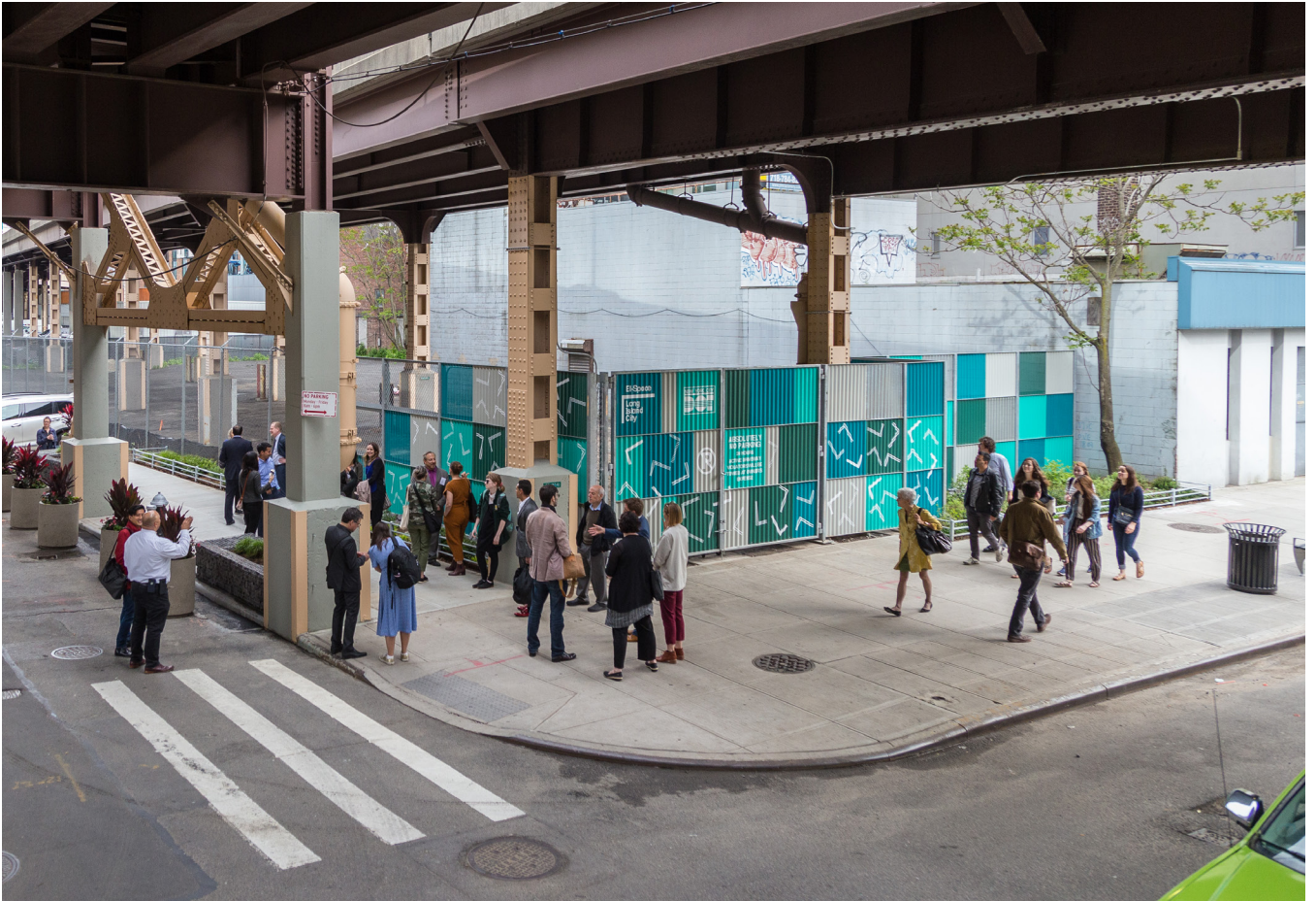
Gabion planters, new sidewalk, and NYC DOT's E1-Fence at Dutch Kills Street and Jackson Avenue in Long Island City, Queens (NYC Department of Transportation)
