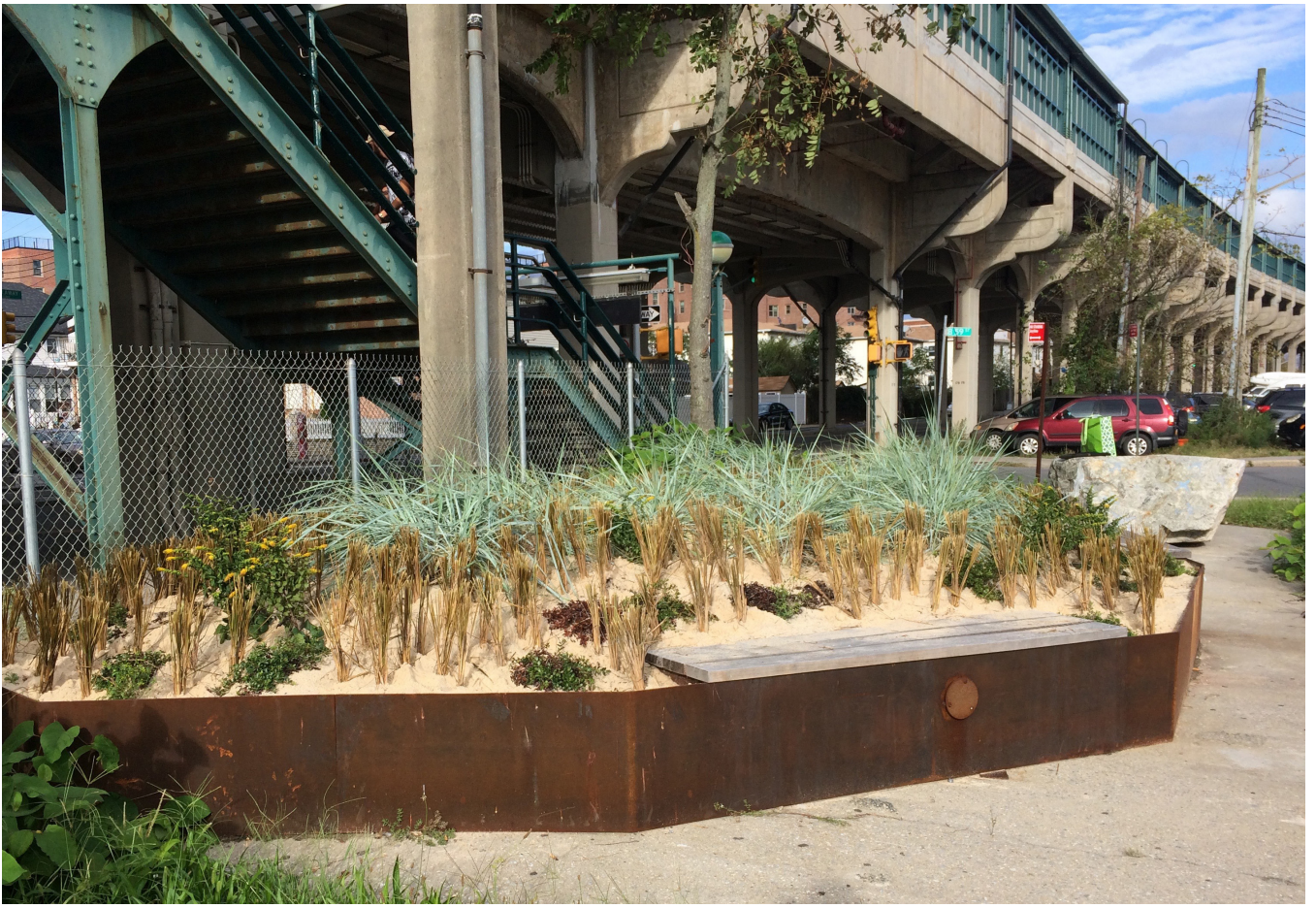
A "dunescape" planter capturing stormwater from the adjacent elevated subway line in Rockaway, Queens (Rockaway Waterfront Alliance)
