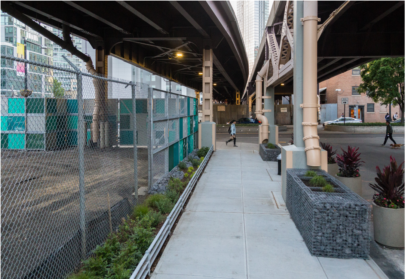
Gabion planters at Dutch Kills Street in Long Island City filtering and slowing down stormwater runoff from the highway above (NYC Department of Transportation)
