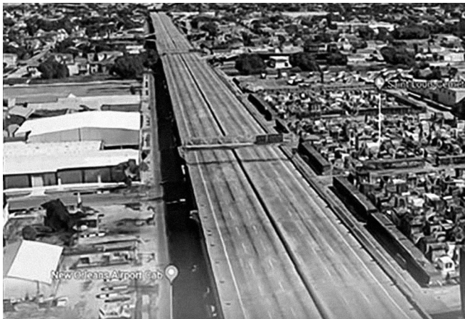
Claiborne Avenue after the construction of I-10 expressway (NOLA.com | The Times-Picayune archive)
